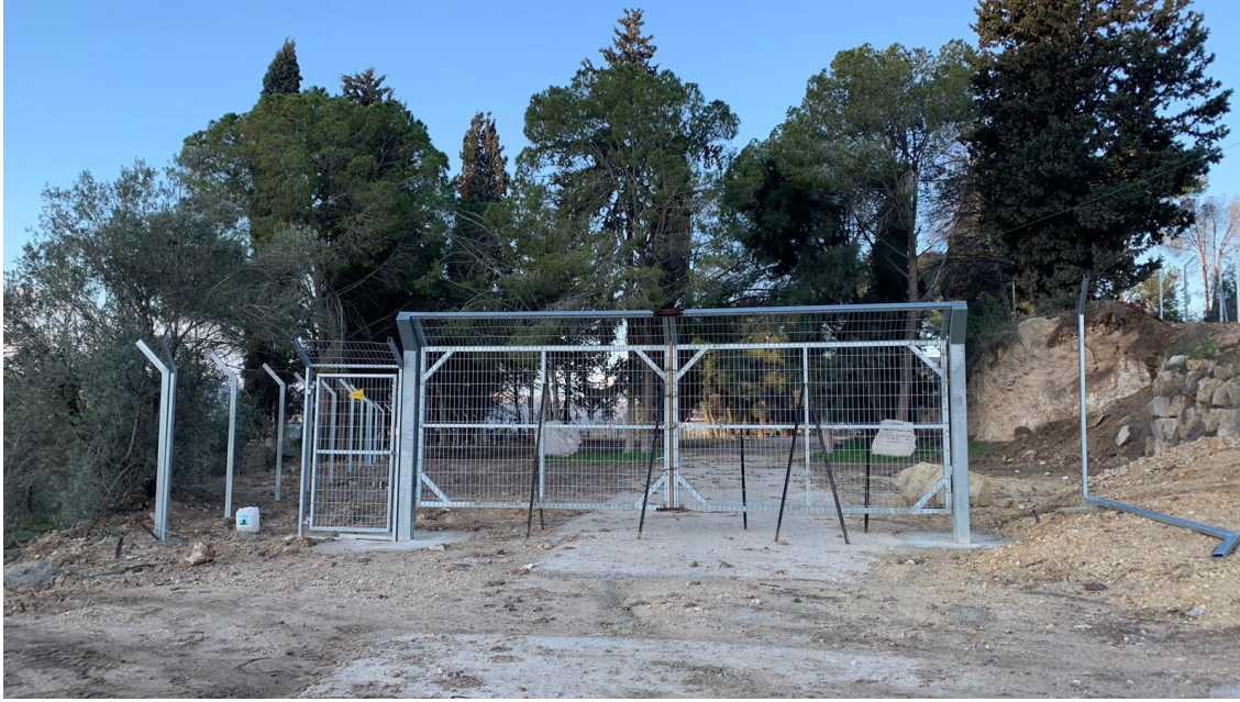
Figure 2: Fence and gate surrounding the Ottoman Hijaz Railway Station buildings in Al-Mas'oudiya
